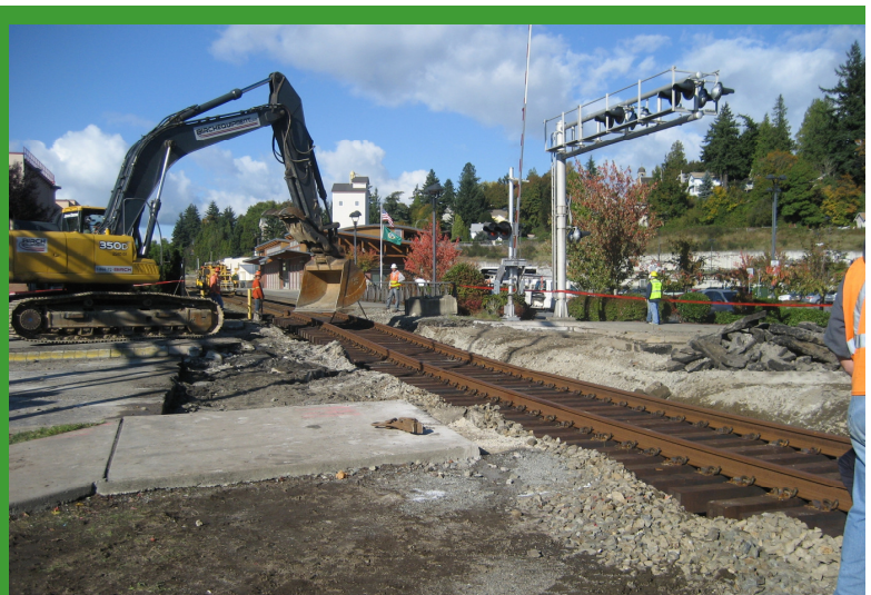
Repairs at Kincaid Street Railroad Crossing
