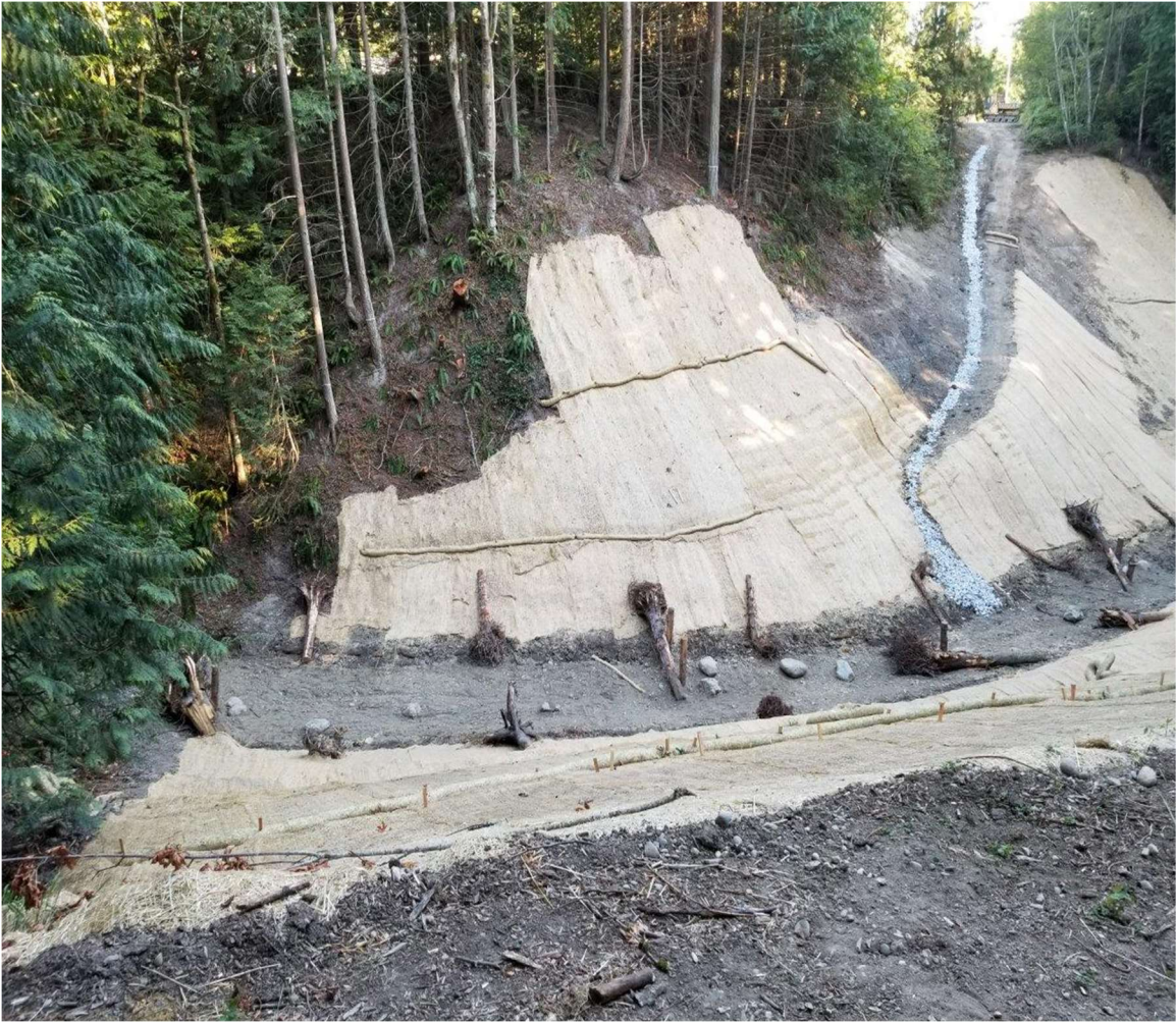
August 2020 Culvert now gone, and new channel opened up.
