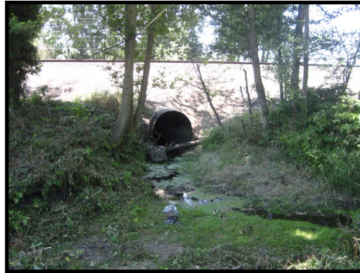
Kulshan Creek City of Mount Vernon/BNSF Bridge Installation Project Prior to Construction
