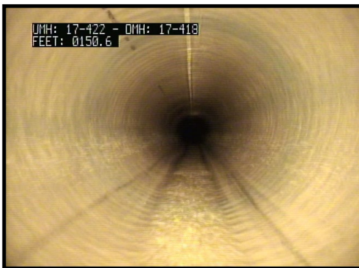
Rusted out CMP after completion of lining
