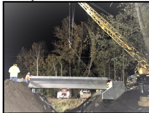
Kulshan Creek City of Mount Vernon/Completed BNSF Bridge Installation Project
