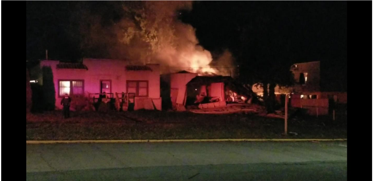
Explosion blew the front of the structure into the front yard and street
