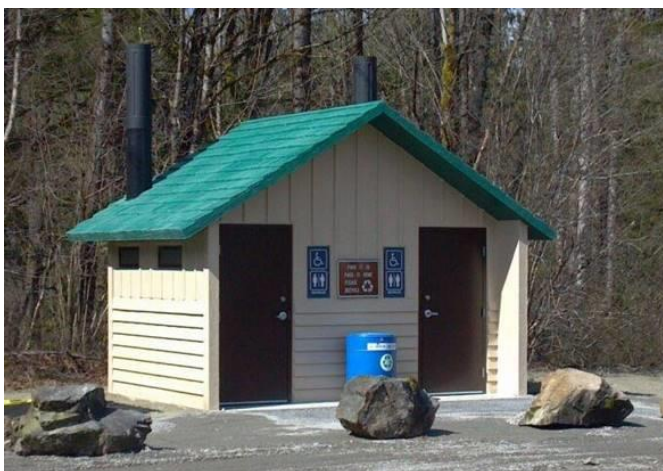
An example of the type of restroom facility to be installed at Little Mountain Park's lower parking lot.
