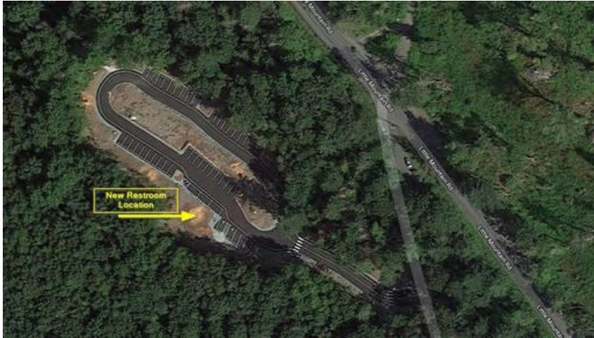
Aerial view of Little Mountain Park's lower parking lot off of Little Mountain Road; as well as the approximate location of the new restroom facility.
