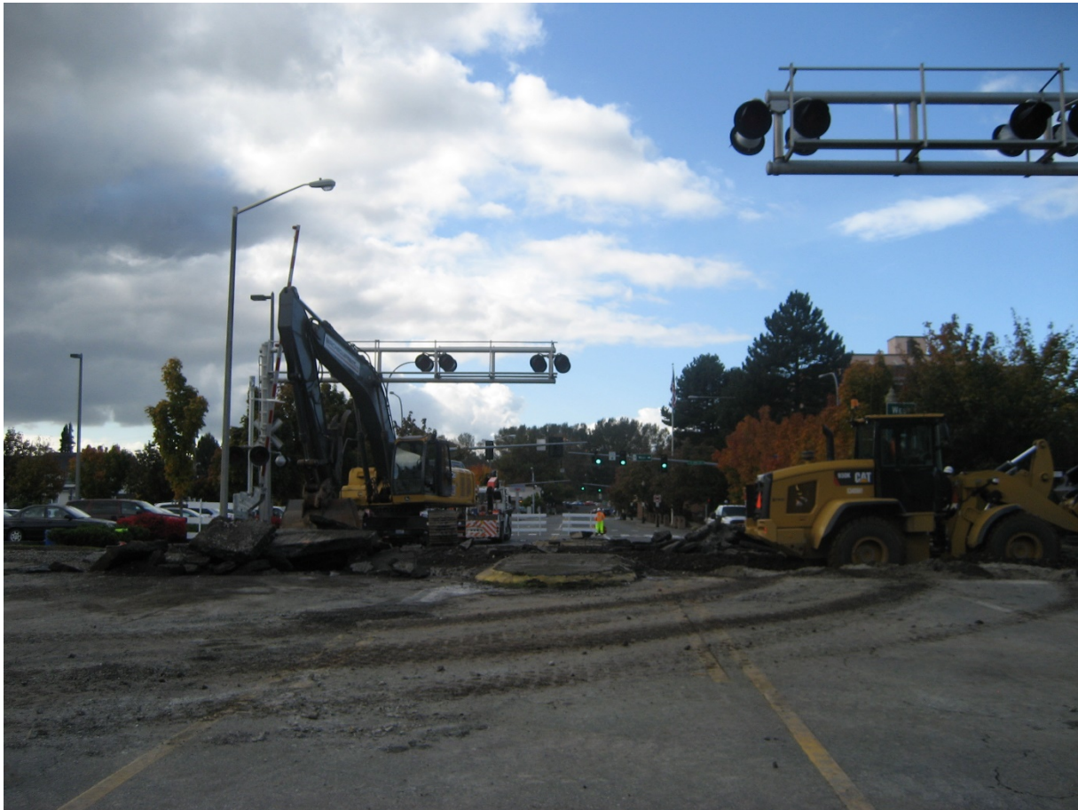
Railroad crossing improvements
