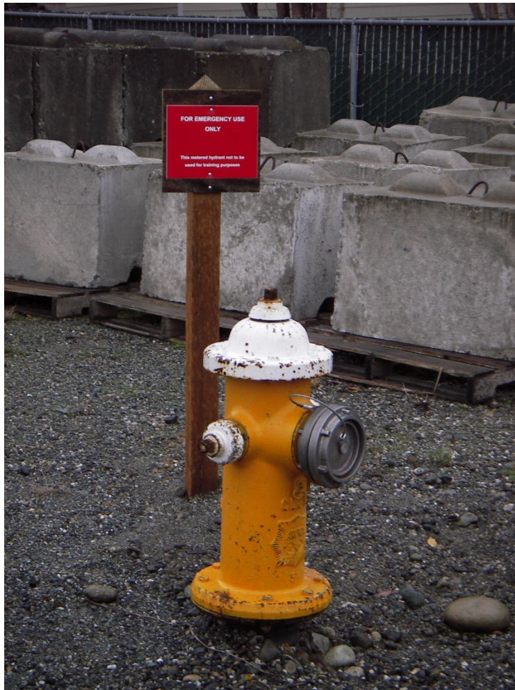
Refurbished Fire Hydrant
