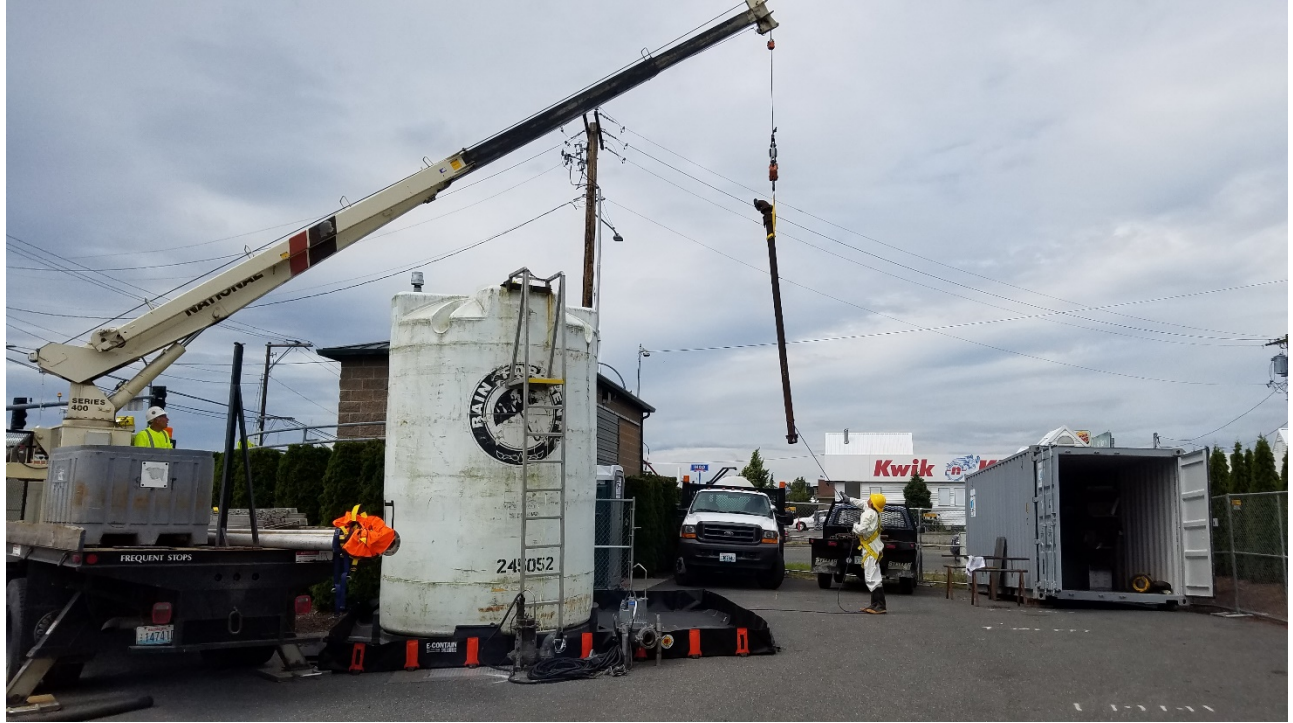
Freeway Drive Pump Station Rebuild
