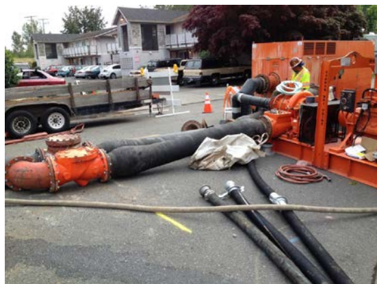
Sewer Lining Project
