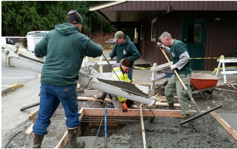
Pouring concrete for the new Hillcrest Lodge Pavilion and BBQ Pit
